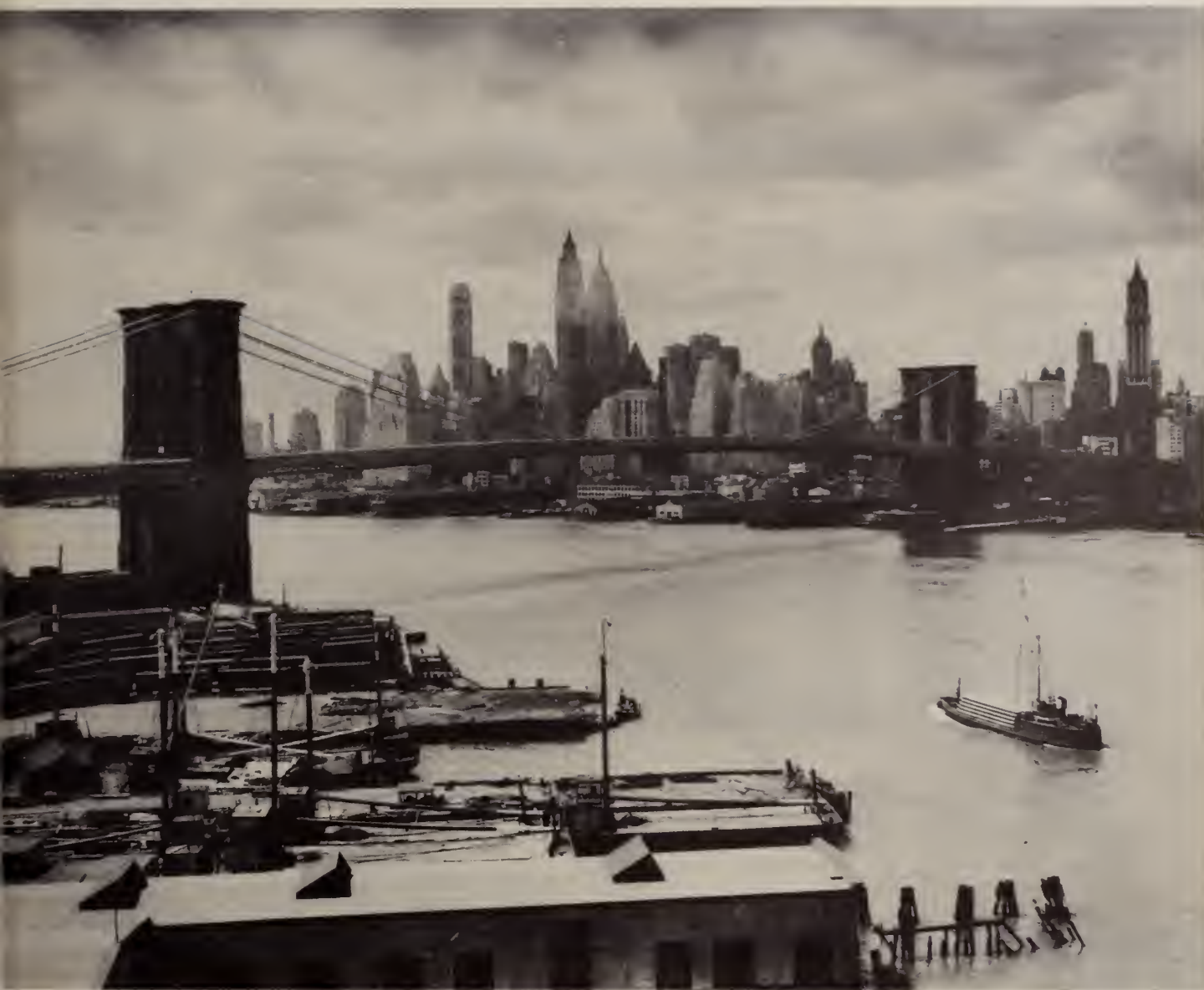
MODERNIZED BROOKLYN BRIDGE , still "a symbol of greatness."
